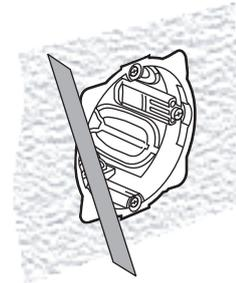
Check that the wall is perfectly flat around the flush-mounting boxes with a ruler or spirit level.
